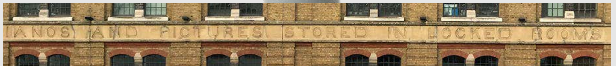
Original retained lettering on exterior of building
